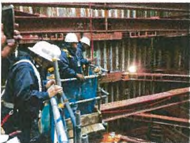
Sewer pipeline construction site
