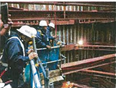
Sewer pipeline construction site
