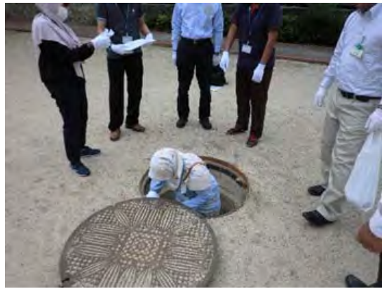
Site Visit at Diversion Manhole (1 September, 2016)
