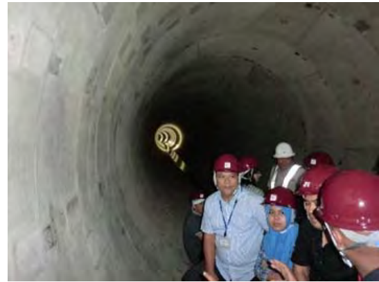
Site Visit at Construction site of Drain laying by Shield Method
