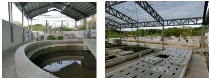
WWTP Construction Project (28 May 2016)
