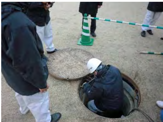
Site Visit at Diversion Manhole (26 February, 2016)
