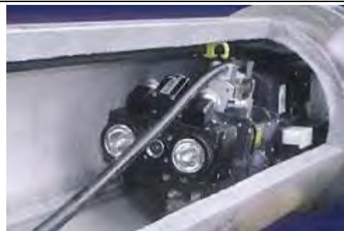
Optical fiber installation
