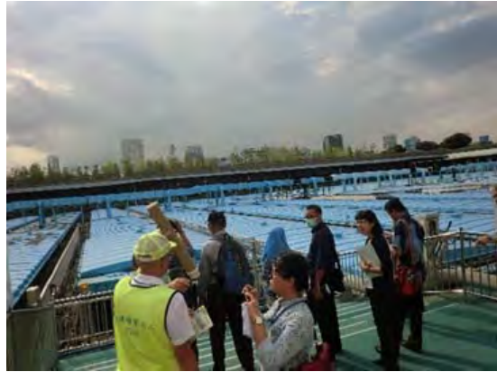
Site Visit at Shibaura Water Reclamation Center (24 August, 2016)
