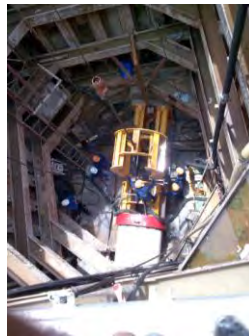
Microtunneling technology for congested road
