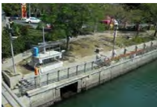
Outlet & Inceptor chamber (Motor-derived gate applied for inflow stop & flood control )
