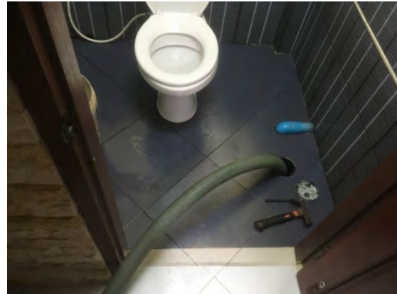
Desludging from Septic Tank
