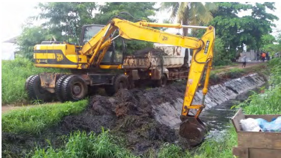
Sludge Removal by Excavator
