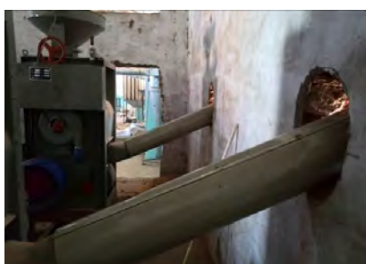
Boring a hole of the duct through the wall. (Northern)
