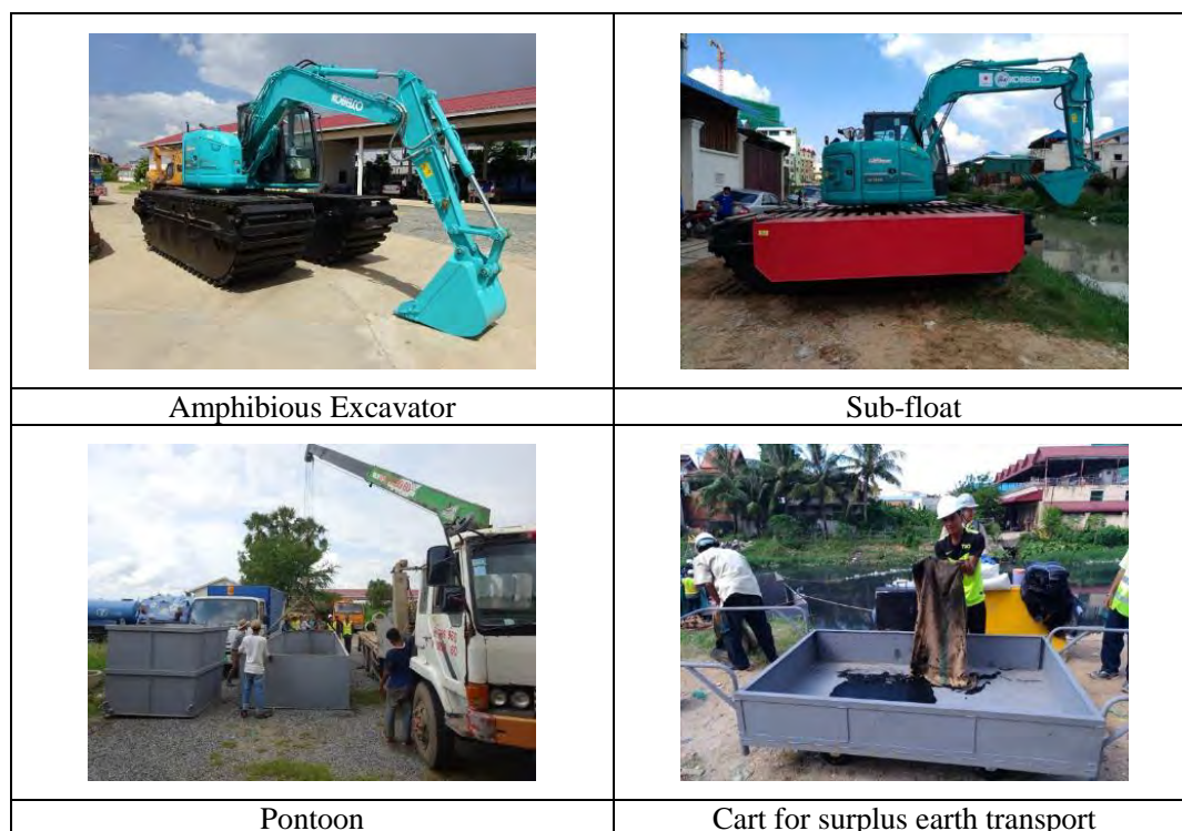
Photo 1 Amphibious Excavator and ancillary facility
