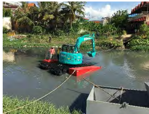
Pull the string that fixes the excavator and set the position
