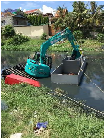
Dredge sludge with bucket
