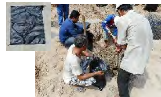
Put the Dried Sludge into Sandbag
