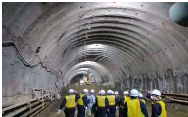
Site survey at SHIN HAKODATE HOKUTO – tunnel construction site
