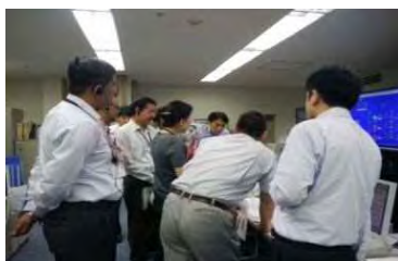
At Monitoring & Control Center of Mechanical Facilities in Tokyo Station (underground)
