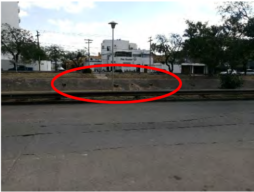
Outlet of Pipe Drainage
