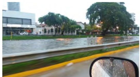
Due to Limited Drainage Capacity
