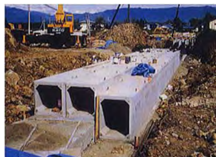
Construction of a Box Culvert Channel below a Public Land
