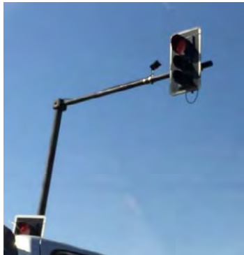
Figure 2.6-16 Traffic detectors to count traffic volume at intersection
