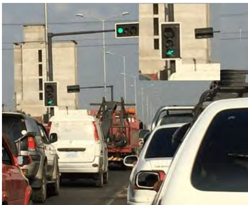
Left turn arrow signal at Av. Virgen De Cotoca Source: JICA study team
