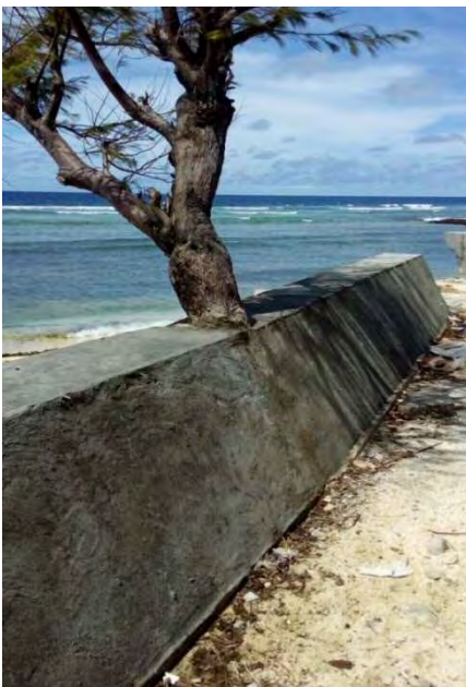
Picture-1 Seawall Constructed by Referring to a Standard Drawing Only (Seawall integrated with base or concrete)
