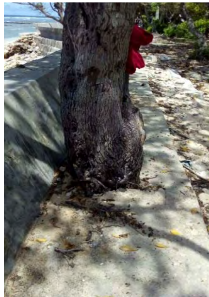
Picture-1 Seawall Constructed by Referring to a Standard Drawing Only (Seawall integrated with base or concrete)
