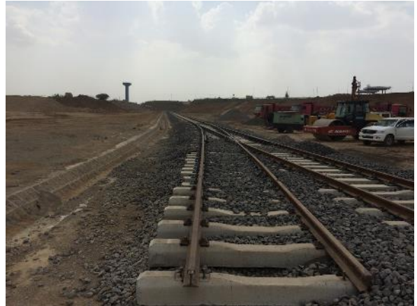
Modjo Dry Port Railway Connection Construction, Ethiopia
