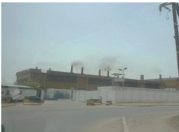
Boulaos Power Station (15 Diesel generators), Djibouti
