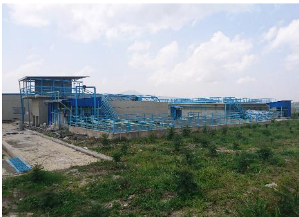
Water Treatment Facility, Bole Lemi Industrial Park, Ethiopia
