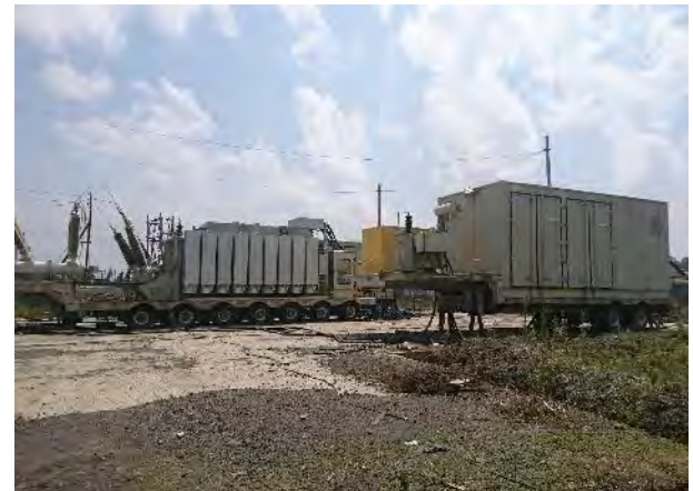
Power Station, Bole Lemi Industrial Park, Ethiopia
