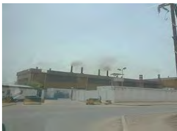
Boulaos Power Station (15 Diesel generators), Djibouti
