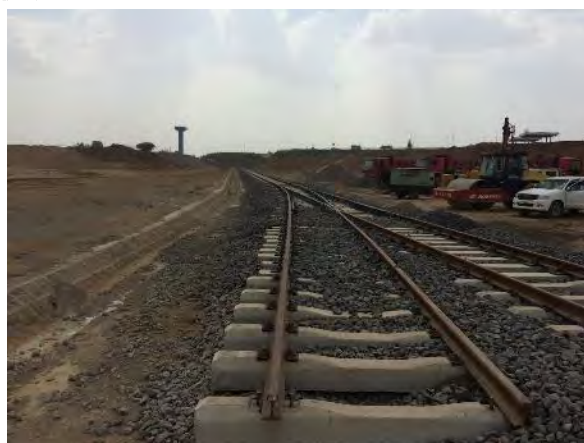
Modjo Dry Port Railway Connection Construction, Ethiopia
