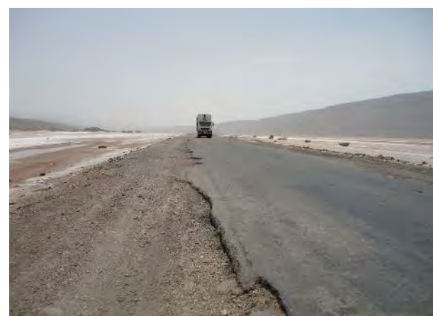
National Route 1 West of Alta, Djibouti
