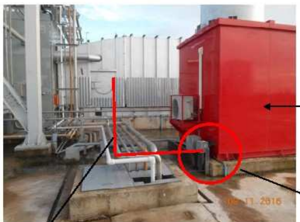
Figure 5.4.2-2 Installation of CO 2 Fire Fighting System Room
