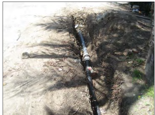
Photo 3-4 Pipe Installation with Shallow Earth Covering
