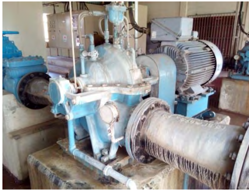
Photo 3-22 Lime Encrust due to Leakage at Pump Shaft
