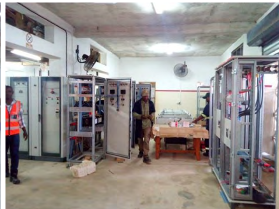
Photo 3-19 Assembling Space for Pump Operator Board
