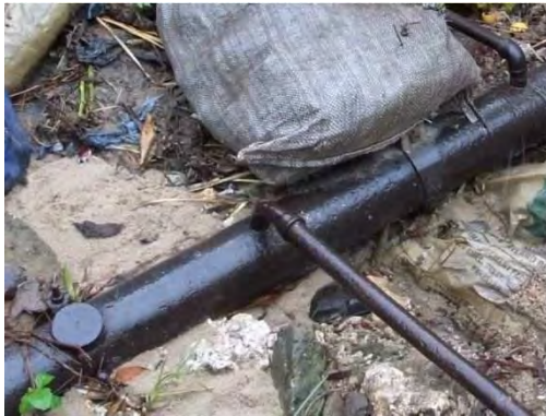
Photo 3-6 Service Connection Branch
