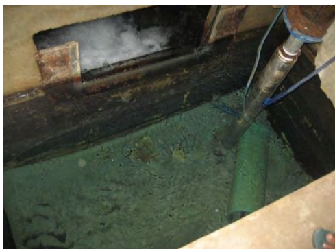
Photo 3-2 Weir Type Flow meter at Bububu Spring
