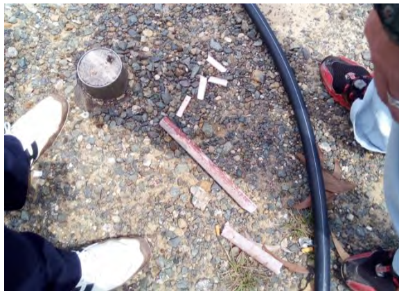
Photo 3-20 Broken Injection Pipe
