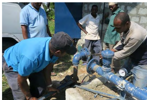
Photo 3-15 Well Pipe Repair
