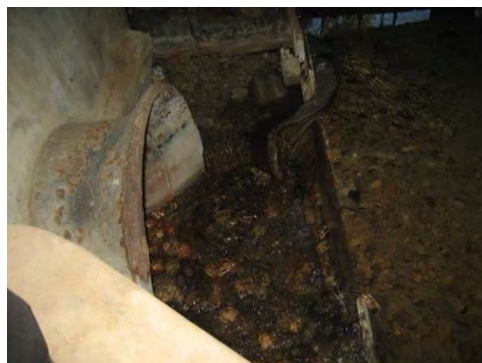
Photo 3-3 Weir Type Flow meter at Mtoni Spring
