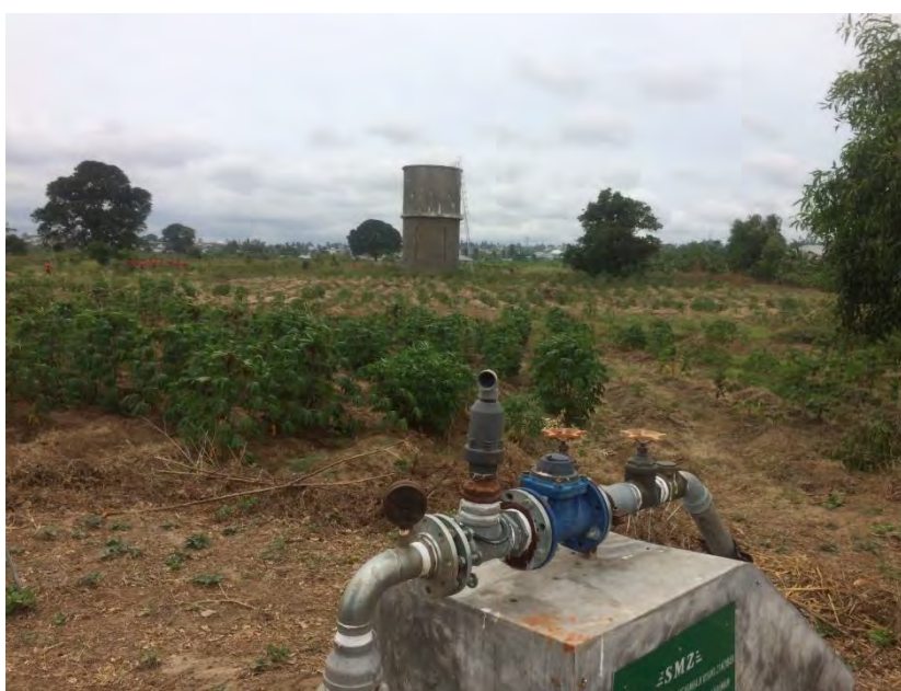
Photo 3-1 Deep Well and Elevated Tank Constructed under Zanzibar Well Drilling Project
