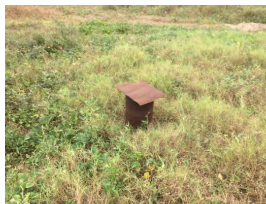
Photo 4-2 Boreholes Developed by Zanzibar Well Drilling Project (Pump not installed)
