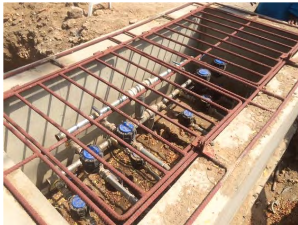
Photo 3-10 Water Supply Facility in Manifold Type in Makadara
