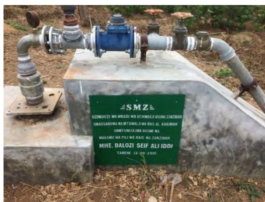
Photo 4-1 Boreholes Developed by Zanzibar Well Drilling Project (Pump is available)
