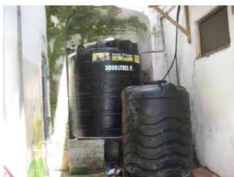
Photo 2-3 Storage tanks of Unofficial Supplier
