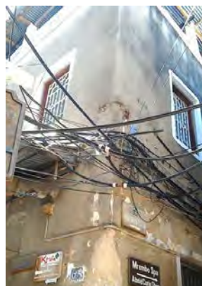
Photo 2-2 Exposed Pipe of Unofficial Supplier (2)
