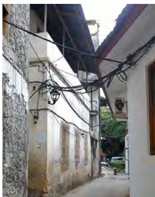
Photo 2-1 Exposed Pipe of Unofficial Supplier (1)
