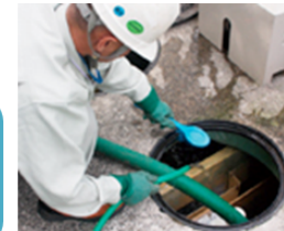
Cleaning of a septic tank
