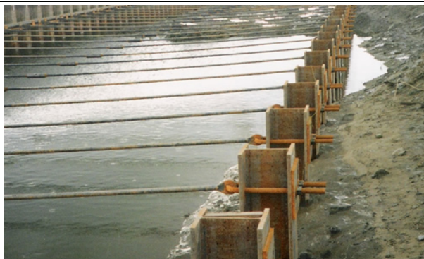
Picture 14-9 Tie Rod and Anchor
