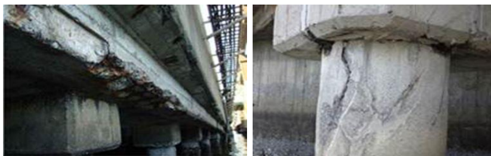
Picture 14-10 Old Concrete Structures Deteriorated by Corrosion
