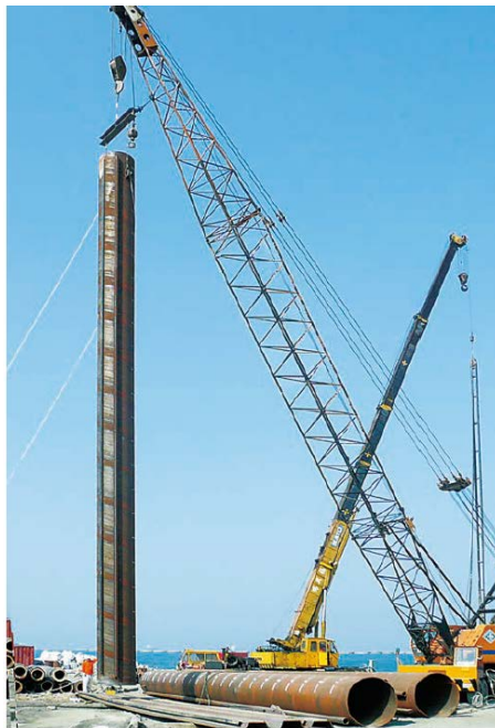
Picture 14-6 Installation of Steel Pipe Pile
