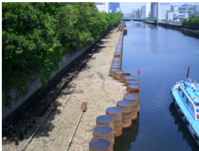
Picture 14-5 Example of Steel Pipe Sheet Pile Method Applied for Seawall
