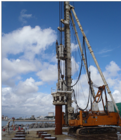
Picture 14-4 Example of Steel Pipe Pile Installation
