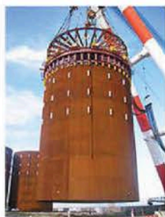
Steel Plate Cellular Shell
