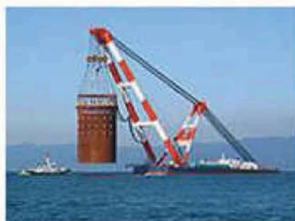
Large Crane Ship
