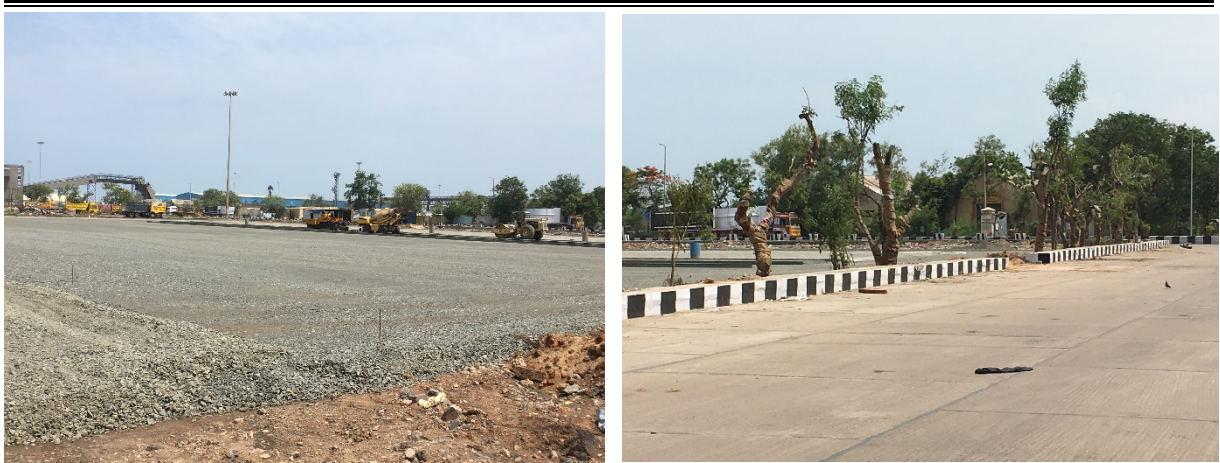
Picture 3-3 Pavement Works and Planting at ONB Area
