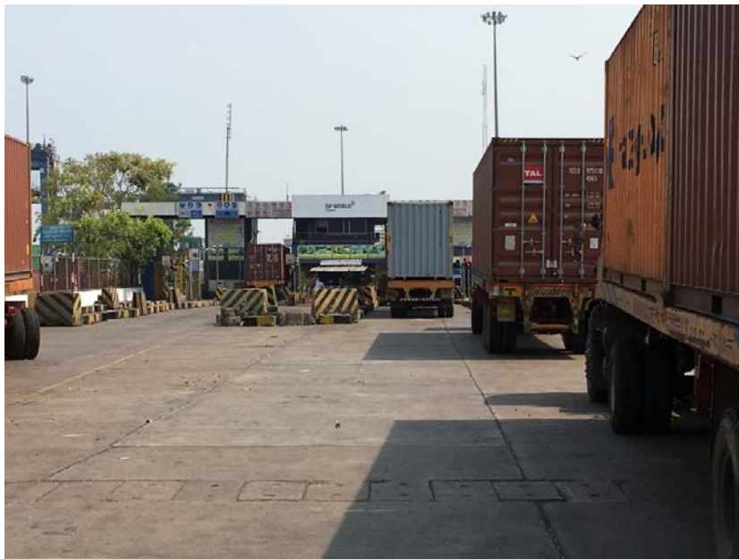
Picture 3-4 Improved DPW IN Gate
