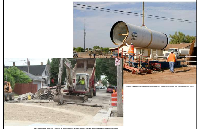
INSTALLATION OF NEW PIPE/ Maintenance of Existing Systems
