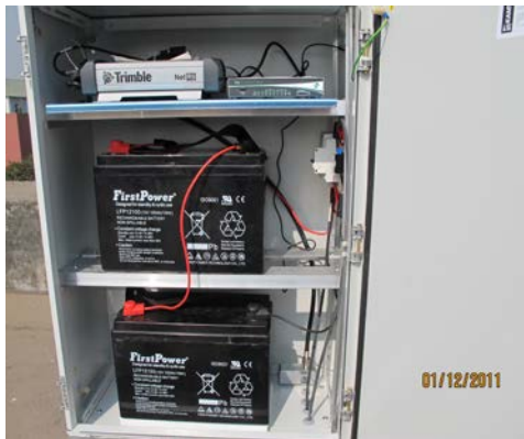
Photo 6.1.3 CORS (inside) (receiver, transmitter and battery)
