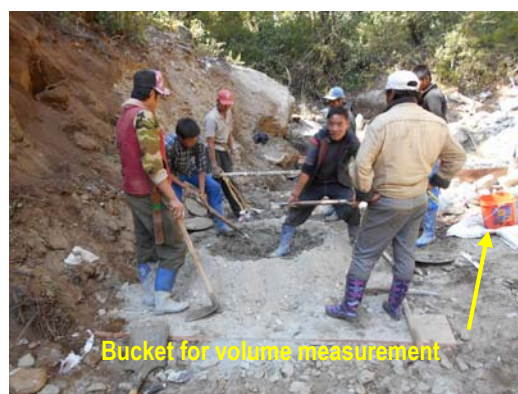
Figure 5.3.17 Concrete Manufacturing Condition
