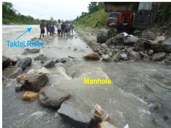
Figure 5.3.3 Water Intake through Manhole
