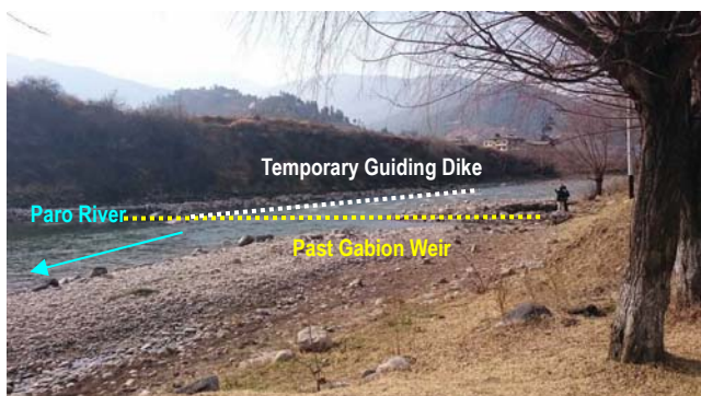
Figure 5.3.9 Past Gabion Weir (Intake Weir-1)
