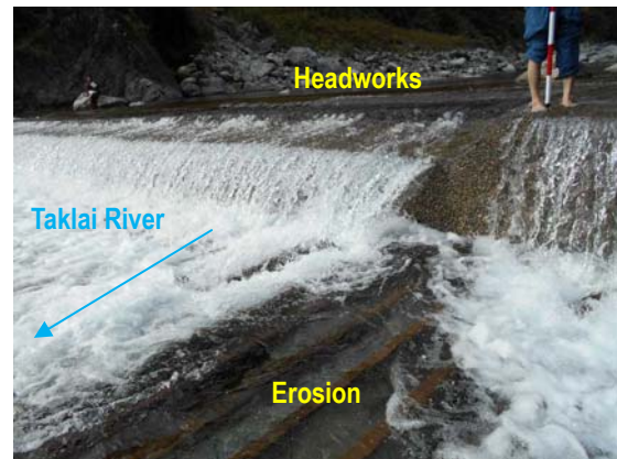
Figure 5.3.4 Erosion on the Apron Concrete
