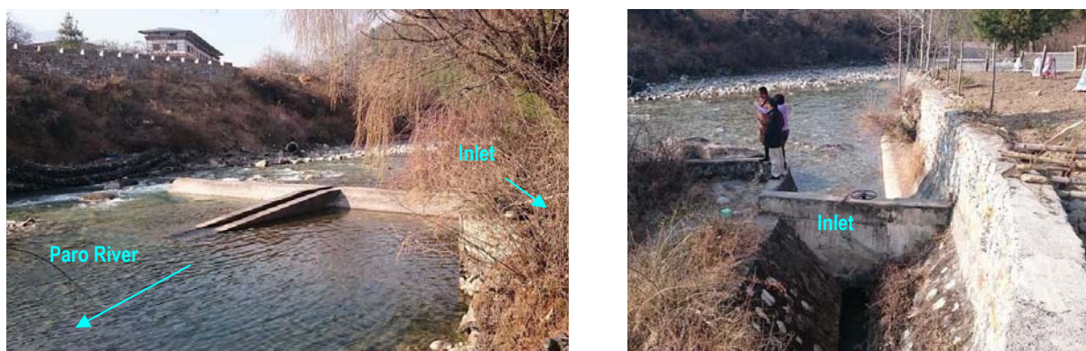
Figure 5.3.12 Weir and Inlet (Intake Weir-3)
