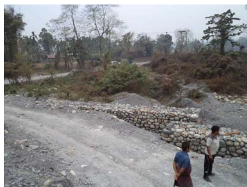
Figure 5.3.10 An Example of Gabion Weir
