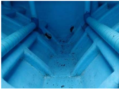
Bottom of the tank before modified
