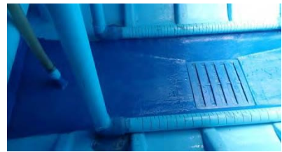
Completion of slope in the bottom of tank
