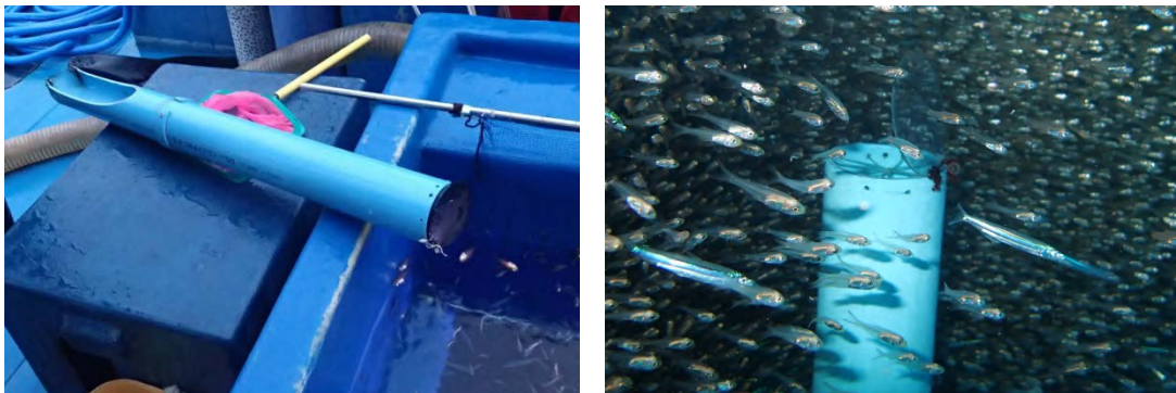
Figure 8: Water intake pipe with check valve
