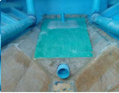
Making drainage pipe from the stern
