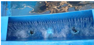
All drainage water come together in one place
