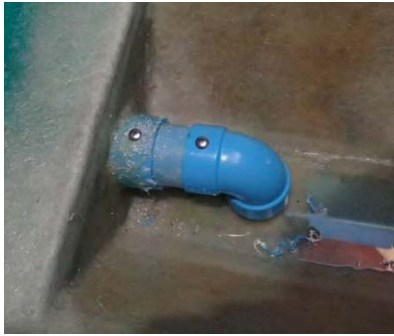
Removable pipe for dead bait drainage
