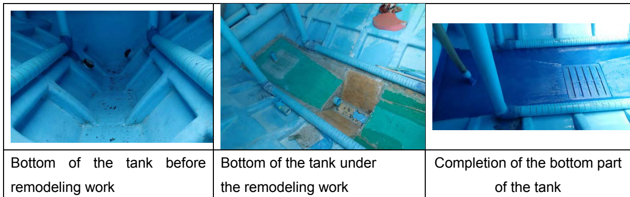
Figure 4: 2nd live bait tank remodeling work
