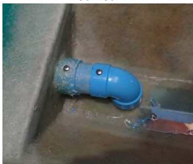
Removable pipe for dead bait drainage
