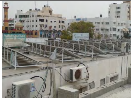
Photovoltaic system of Shifa Hospitals
