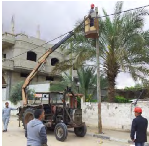
Figure 2-9 Dangerous elevated work with a bucket truck (without a safety belt and outrigger)
