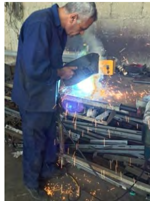
Black smith of transformer repair
