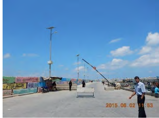
Street lighting with Photovoltaic system of Gaza Port
