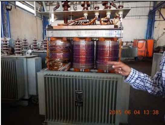
Transformer repair factory
