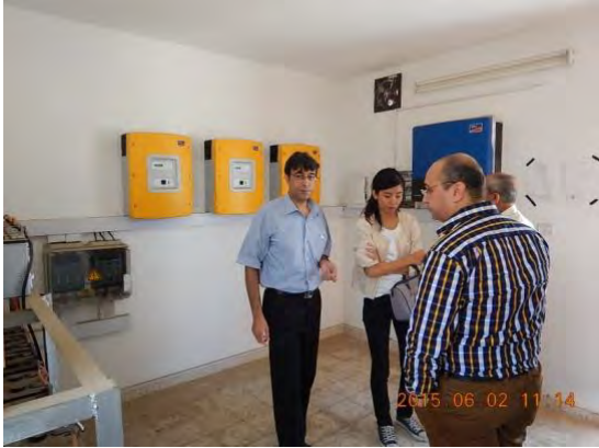
Photovoltaic system of Al Faloja School
