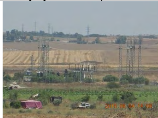
Gaza North Substation (Construction is suspended)
