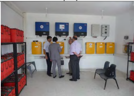
Photovoltaic system of Shifa Hospitals
