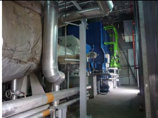
Repaired generator of Gaza Power Plant
