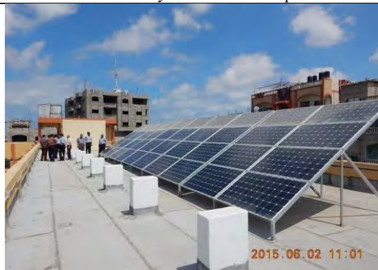
Photovoltaic system of Al Faloja School
