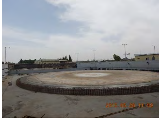
Foundation of Gaza Power Plant (Construction is suspended)
