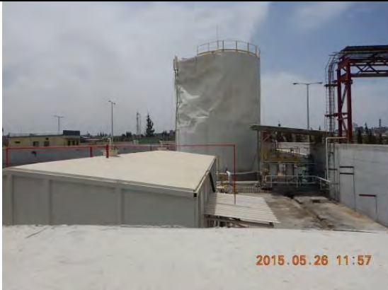
Temporary fuel tank of Gaza Power Plant (The building of lower left)
