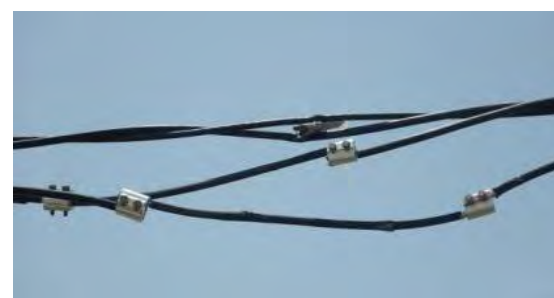
Figure 1-17 Temporary repair using PG clamps
