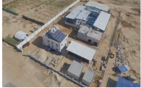
Sea Water Desalination Plant Site Supported by UNICEF (Capacity 2,000m 3 /day)
