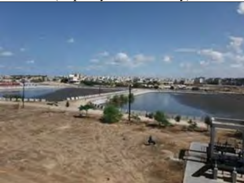
Anaerobic Lagoons in Rafah STP
