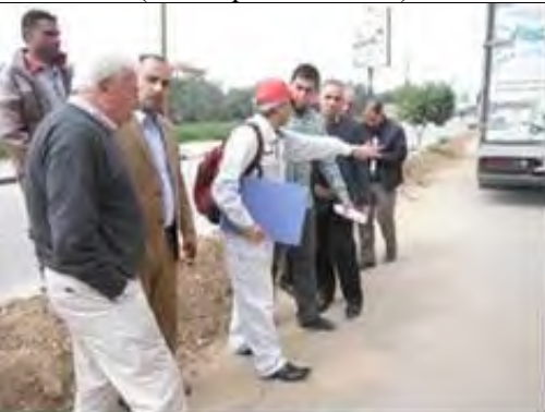
Construction Supervision for the Pilot Project in Absan Al Kabera (7 th March 2017)
