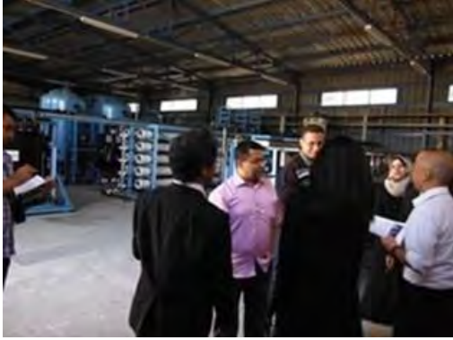
Sea Water Desalination Plant Supported by ADC (Capacity 600m 3 /day)
