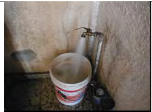
Confirmation of water supply improved by the Pilot Project in Rafah (8 th March 2017)
