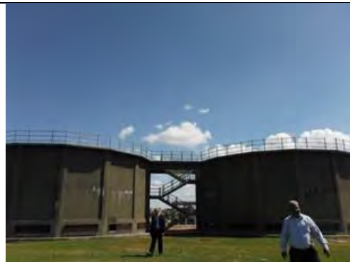
Trickling Filters in Rafah STP
