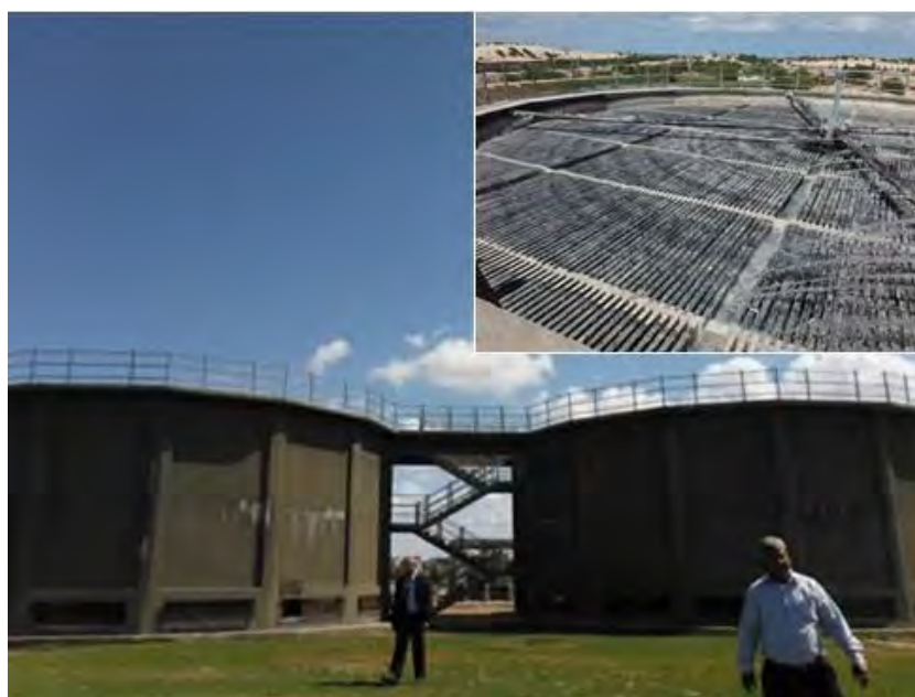
Photo 6-1 Trickling Filters installed in Rafah WWTP and its Top Part
