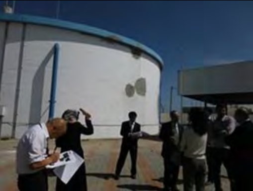
Water Reservoir Supported by IsDB (Capacity:3,000m 3 )
