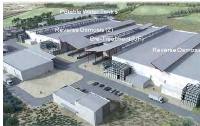
出典: European Investment Bank Group, Gaza Central Desalination Plant Project “The Impact on Water Security in Gaza” August 2016
