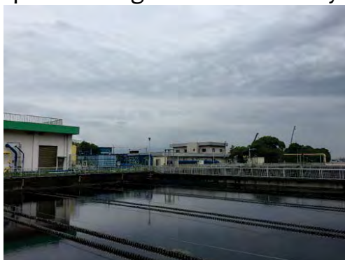
Sedimentation tanks
