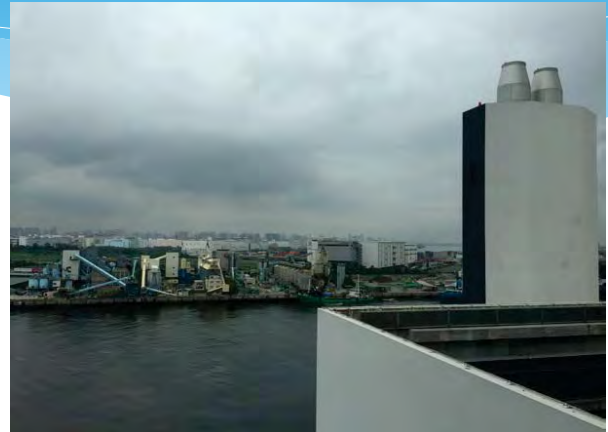
Chimney after the burning process
