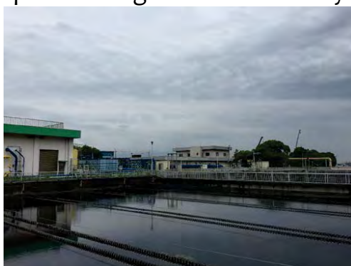
Sedimentation tanks
