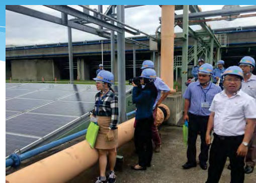
Solar panels cover reaction tanks
