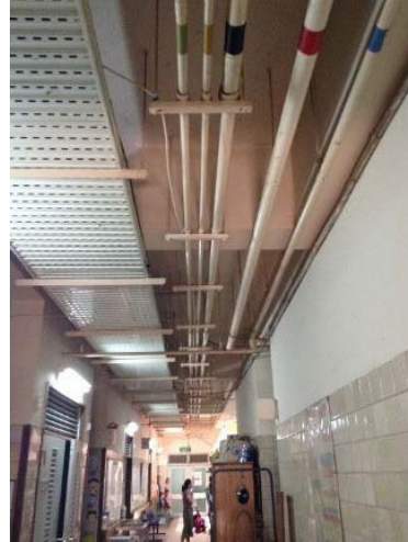
Photo2-3 Exposed Pipes of Medical-Gas (O 2 , compressed air, vacuum)
