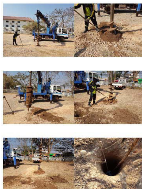
Photo 1-2 Test-drilling Hole BH-1
