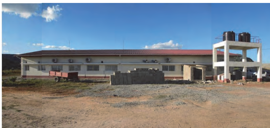
After Completion Taken from South, 2nd July 2015
