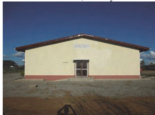
After Completion Taken from West, 2nd July 2015
