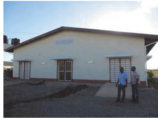
After Completion Taken from East, 2nd July 2015
