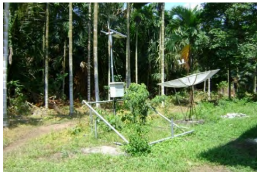
Telemetry-based Peatland Water Table Monitoring Equipment made by BPPT MORPOLAGA (Sanggar Seni, Public Accommodation of Sub-district Office in Des. S. Tohor, Sub-district Tebing Tinggi Timur, Kepulauan Meranti District, Riau Province ; 17 Jul. 2017)
