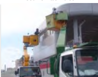
Toll Booth Facilities
