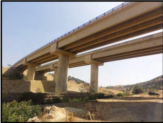
(1) EELKELL Bridge (July 10 th , 2017 – July 15 th , 2017)
