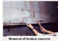
Removal of broken concrete
