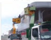
Toll Booth Facilities
