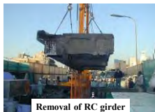
Removal of RC girder
