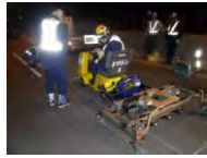
Fatigue Damage Detection Device of Orthotropic Steel Deck
