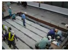
Removal of RC girder
