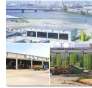
Tunnel soil recycling project
