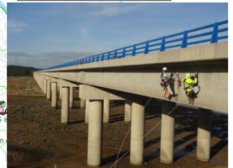
Oued Tahadart Bridge
