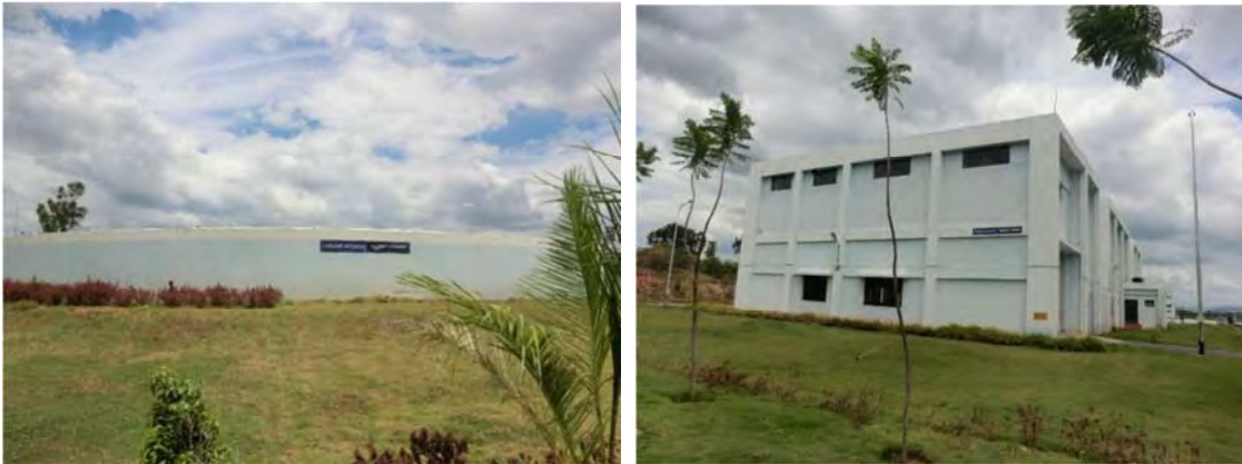
Photo 14.2.2 TK Halli WTP with Pump Station
