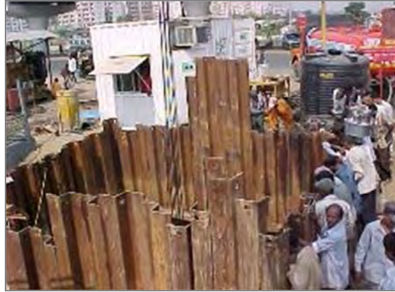
Photo 12.2.3 Trenching with Sheet Piling
