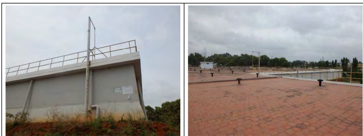
Photo 12.1.8 Current Status of Existing GKVK GLR
