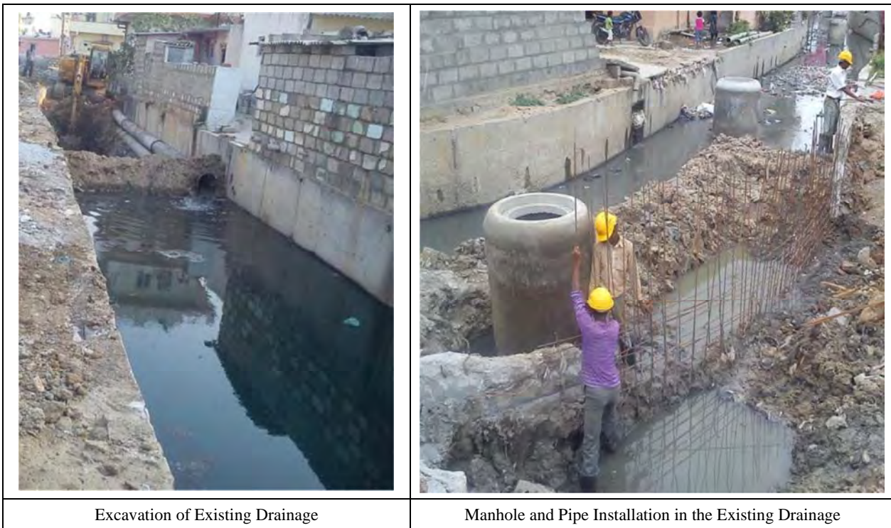
Photo 10.2.21 Installation of Sewer Line under Drainage Bed
