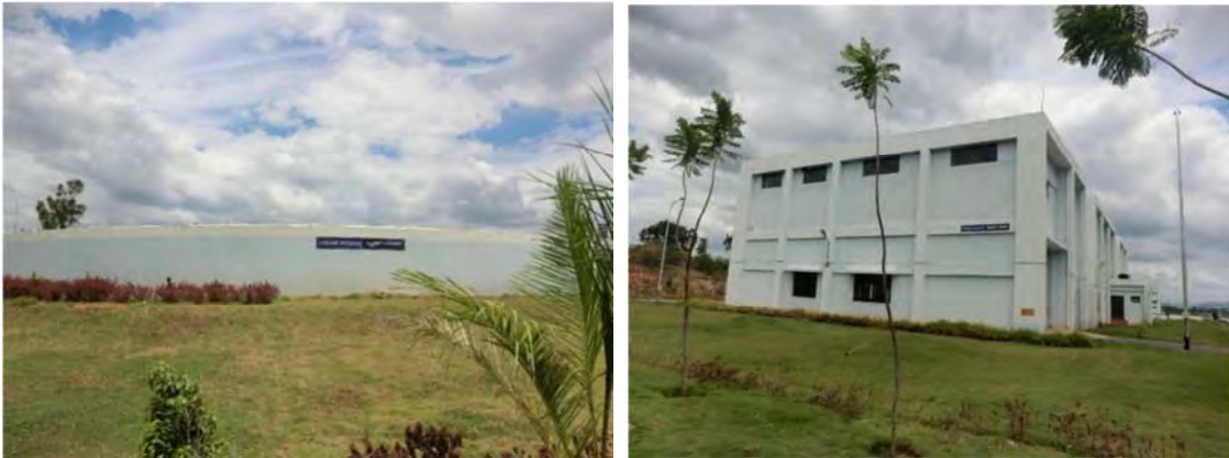
Photo 14.2.2 TK Halli WTP with Pump Station
