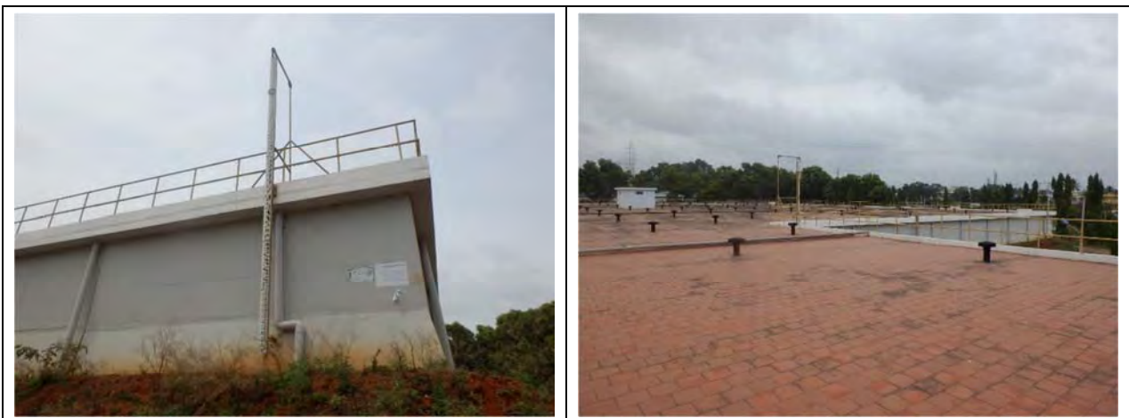
Photo 12.1.8 Current Status of Existing GKVK GLR
