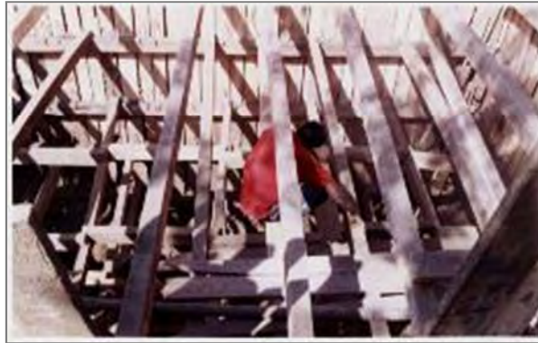
Photo 12.2.1 Conventional Trenching Method
