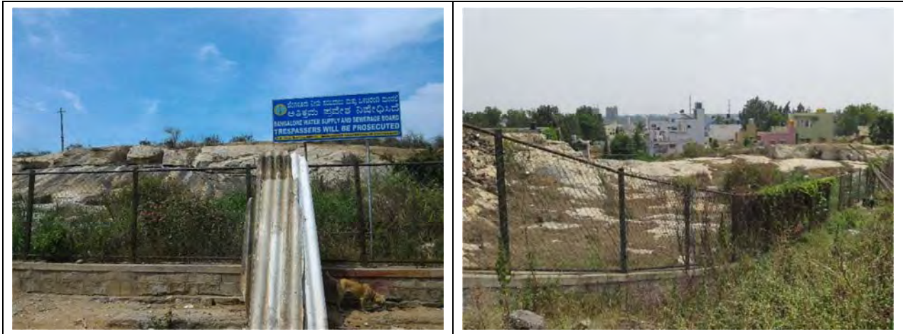
Photo 12.1.1 Current Status of Proposed Land for the construction of Gottigere GLR
