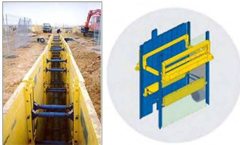
Photo 12.2.2 Trenching with Trench Boxes
