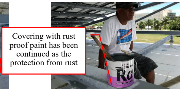
Coating of Rust Proof Paint
