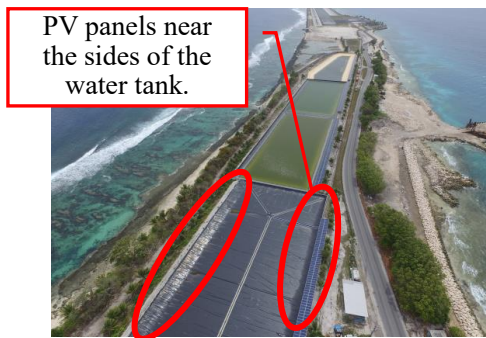
The PV Facilities near the sides of the water tank
