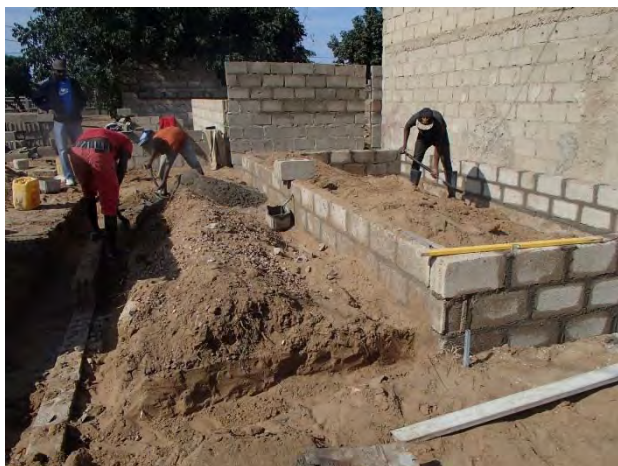
Facility Installation Work
