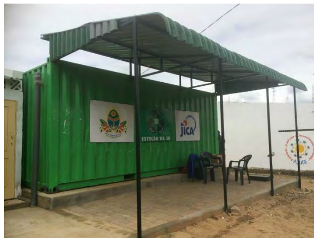
Installed Valuables Recovery Facility (3R Station)
