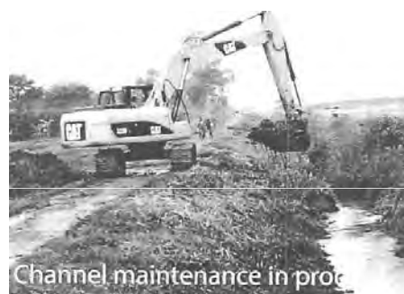
Sample image of de-silting (twice in a year) from main canals at the Doho Rice Irrigation Scheme in Butaleja District (source: DIFACOS).
