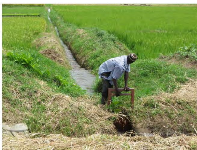
Water gate at secondary canal to tertiary canal (Doho Irrigation Scheme)
