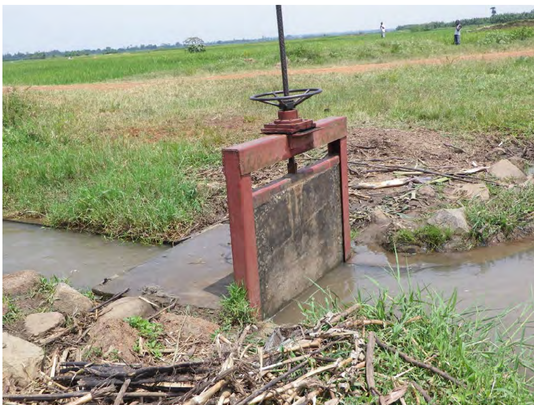
Water gate at the main canal (Doho Irrigation Scheme)
