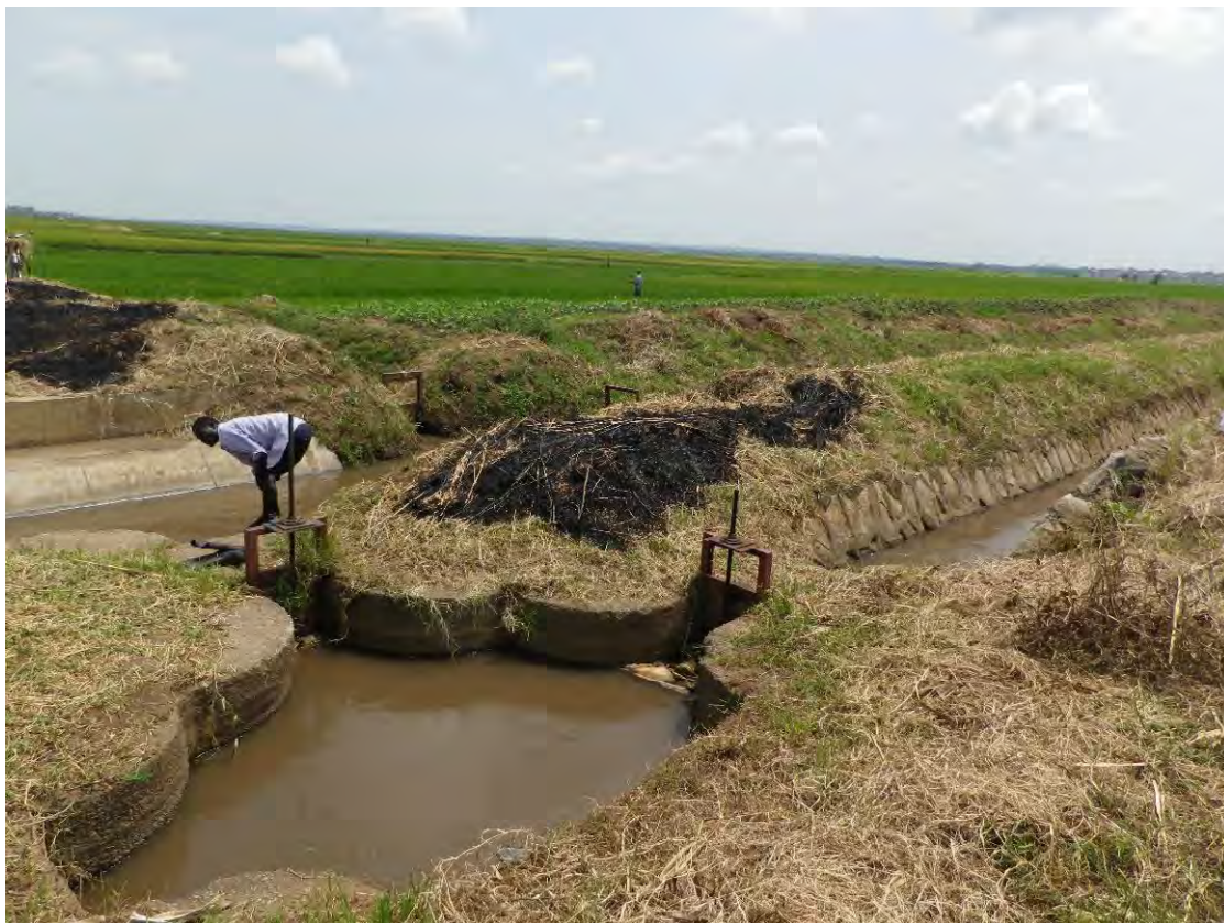
Diversion of water and water gate at the secondary canal (Doho Irrigation Scheme)
