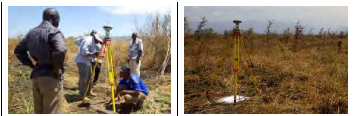
Figure 1.6 GNSS Observation Work
