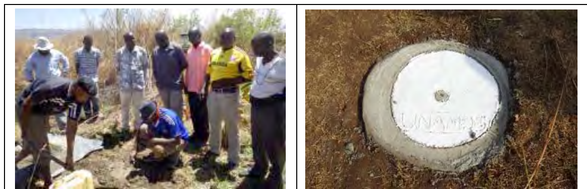
Figure 1.4 Monumentation work and Monumented GCP
