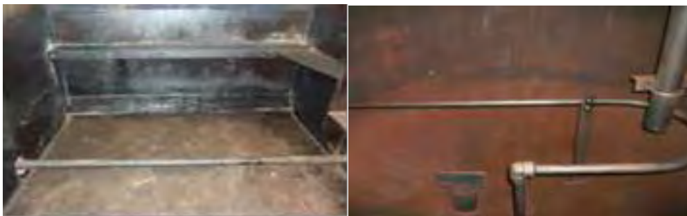
Figure 11-33 Image of fuel tank before and after cleaning by MDS
