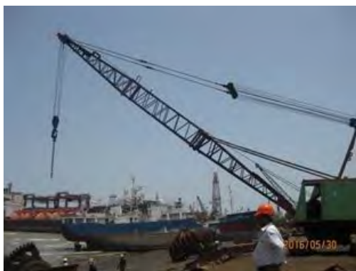
P.68 75 tons Crane
