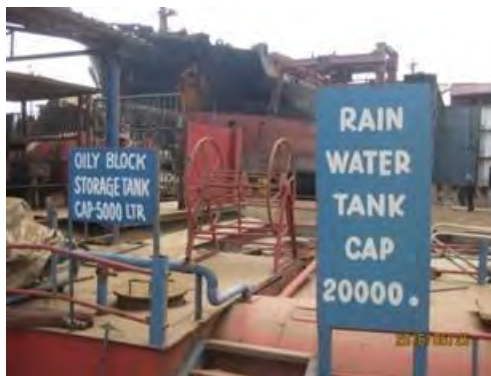
P.78 various tanks
