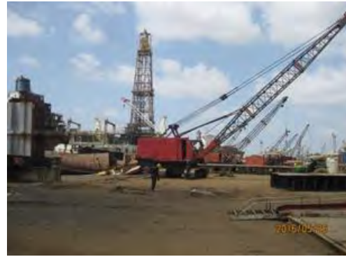
P.78 many cranes are working along the shore line
