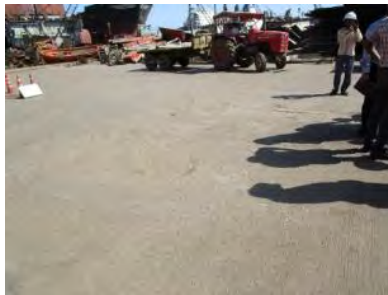
Concrete floor on the yard (NK certified yard)
