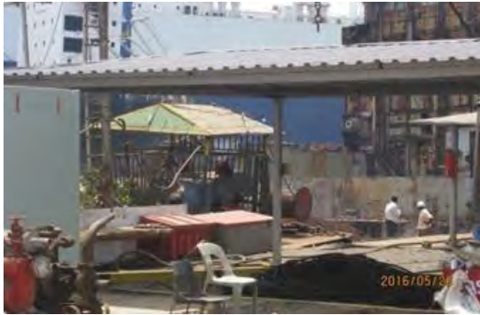
P.5 wire storage space with roof behind a winch
