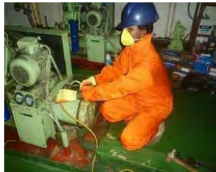
P.V-7 collecting freon gas (phot provided by yard)
