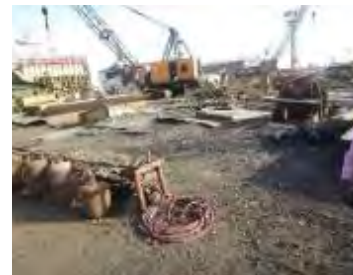
LPG is stored close to cutting zone (Normal yards)
