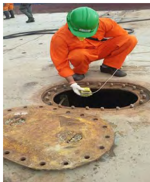
Confirmation on gas content in closed spaces (yard in process of verification)
