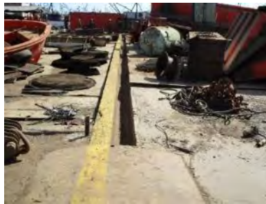
Drainage pit to prevent pollution on the soil and sea (NK certified yard)
