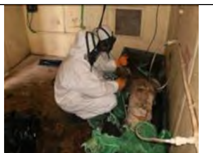
Asbestos removal by mobile contamination unit (All yards)
