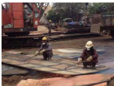
Proper PPE during gas cutting (NK certified yard)
