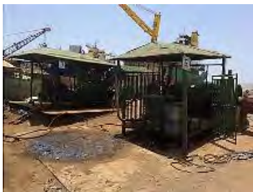
Fence around the winch for safety (All yards)
