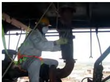
Wearing safety belt during working at height (NK certified yard)
