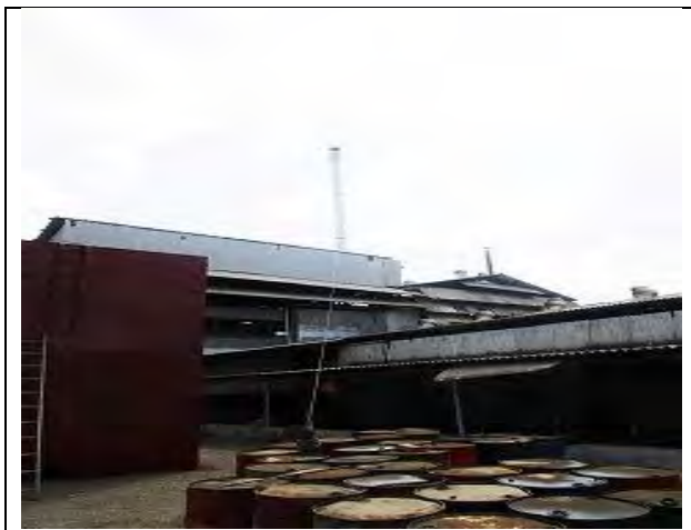
Refinery of Used Fuel oil (Main Building)
