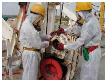
Asbestos removal on board (NK certified yard)
