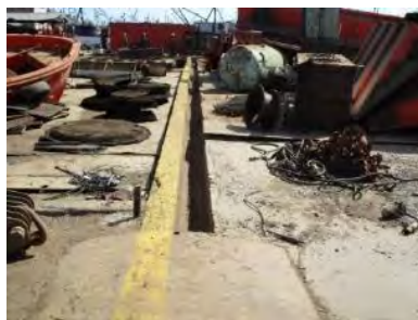
Drainage pit to prevent pollution on the soil and sea (NK certified yard)
