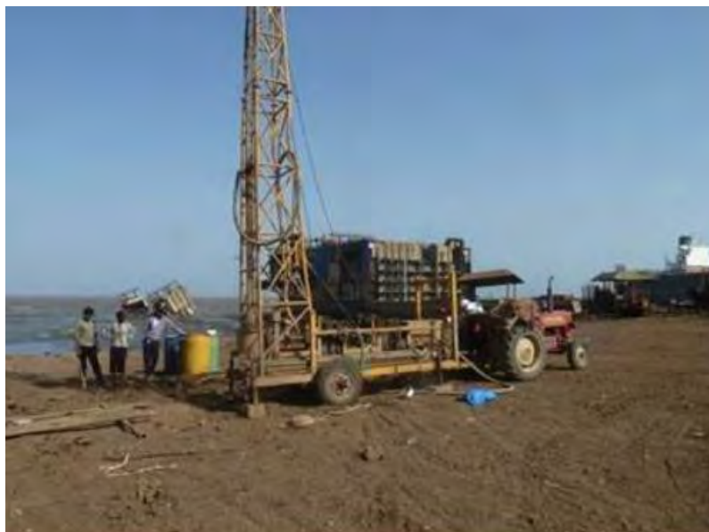
Figure 3-6 Boring at Seashore
