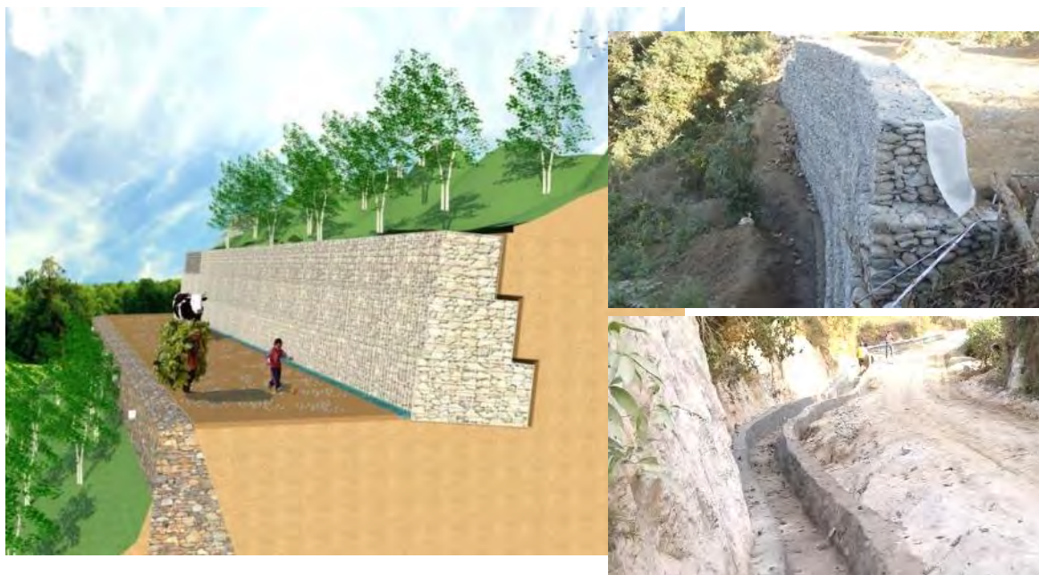
Figure. 4.3 Recovery of Road Facilities with Retaining Wall, Side Drains and Cross Drains in Bhotechaur (Melamchi Municipality), Sindhupalchowk
