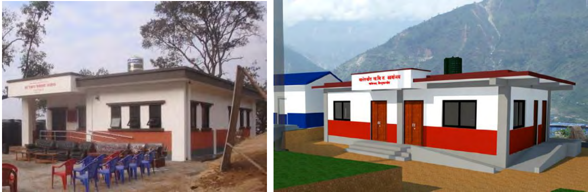
Figure. 4.1 Recovery of Social Services and Development Activities through the Reconstruction of VDC Building in Thokarpa VDC (Left) and Maneshwara VDC (Right: Ongoing)
