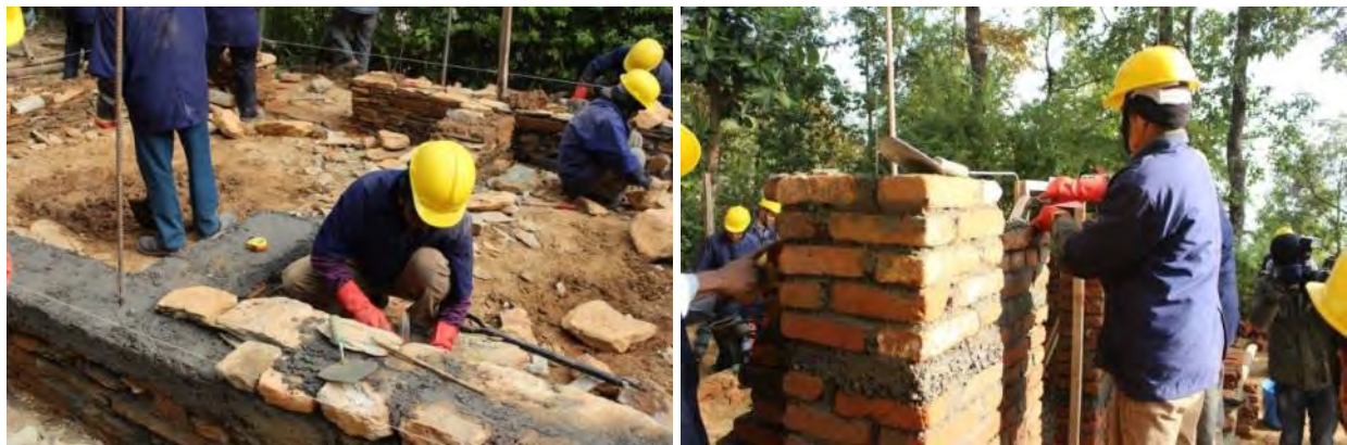
Source: JICA Project for the Transitional Project Implementation Support for Emergency Reconstruction Projects Picture 2.1 House Reconstruction Training for Masons
