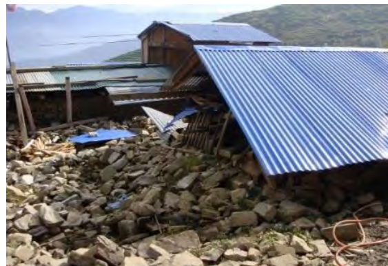
Picture 3.4 Collapsed House (Laprak)
