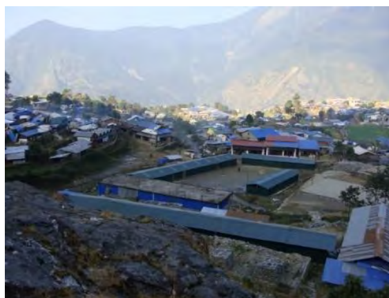
Picture 3.6 Temporary School Building at Barpak
