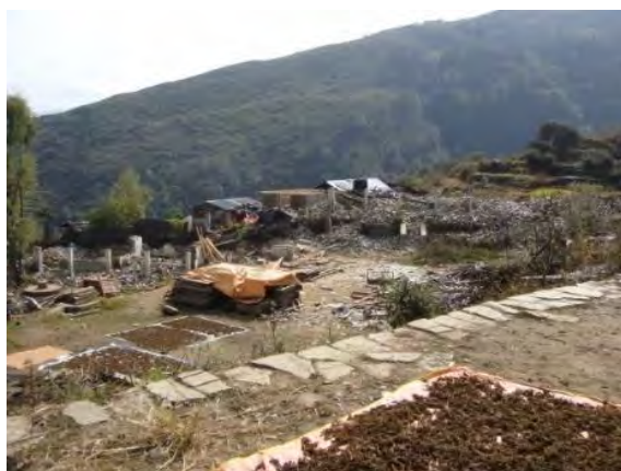
Picture 3.5 Collapsed School in Laprak
