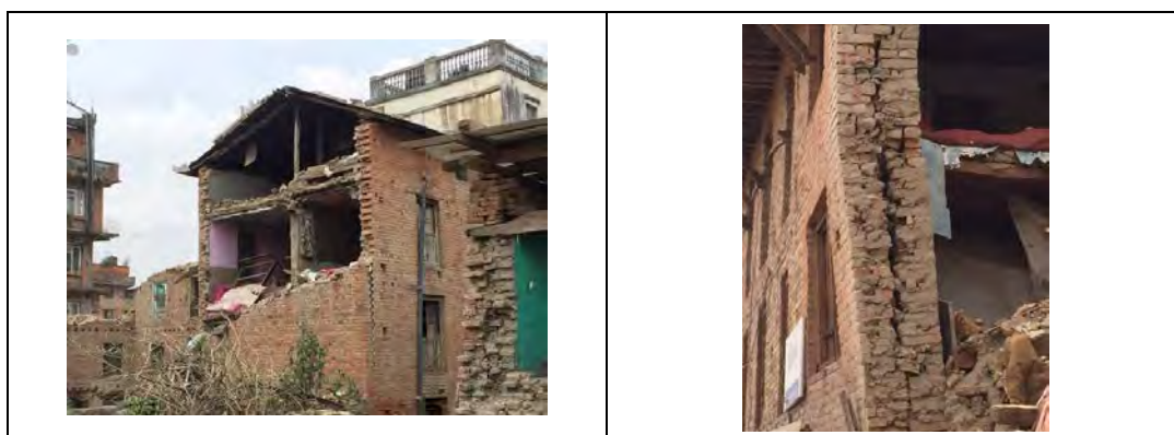
Figure 8.2.4 Out-of-plane Behaviour and Delamination of Walls
