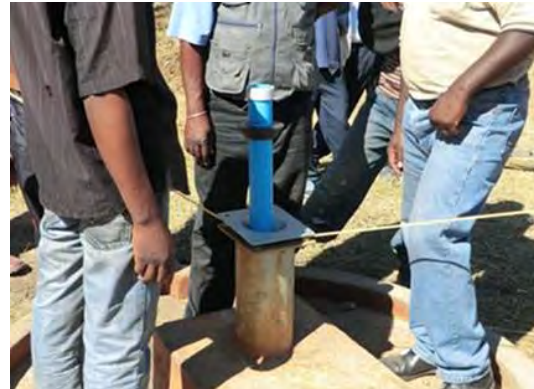
Replacement with PVC riser pipes (Afridev hand pump)
